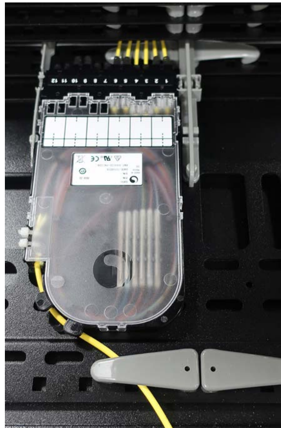
Figure 22. Installing Cassette in CHD Panel
