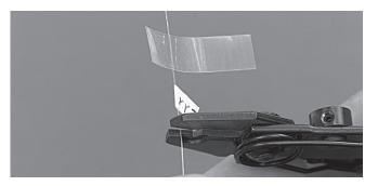
5.3 Select the appropriate fiber to be spliced, cut the identification flag when available and do all necessary steps till the splice protector is installed.
