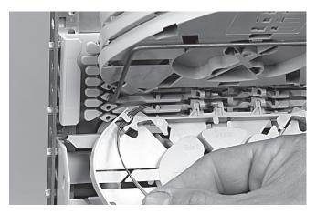
4.7 Pull gently on the fibers in the tray and make sure that the fibers are well contained in the routing block and wraparound groove plate.
