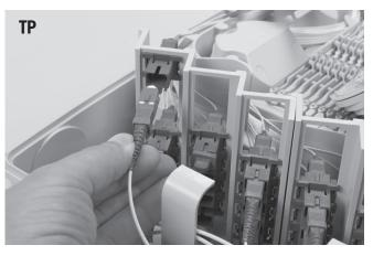
7.2 Once the top row of pigtails is installed, the pigtails can be routed towards the pigtail seal. Insert one by one into the groove.
