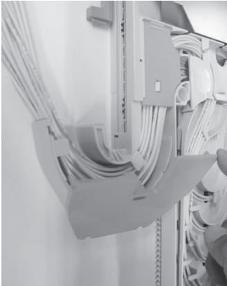
6.3 Carefully close FACT back lid and bend control cover.
