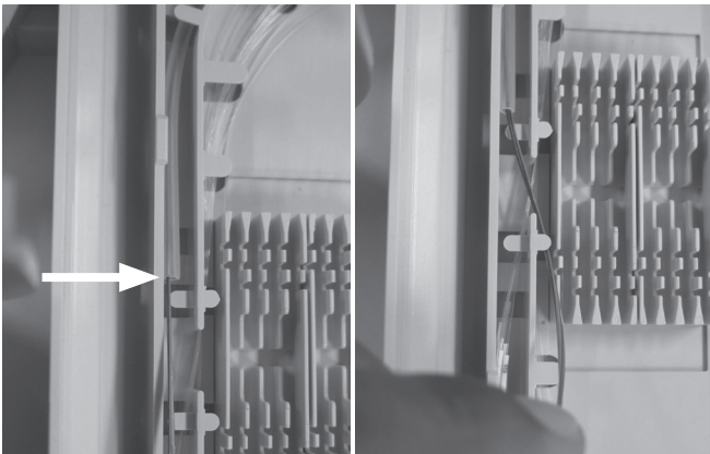
1.7 Stop the overtube at the position (straight area) shown in the picture and guide fibers through the channel into the splicing area.
