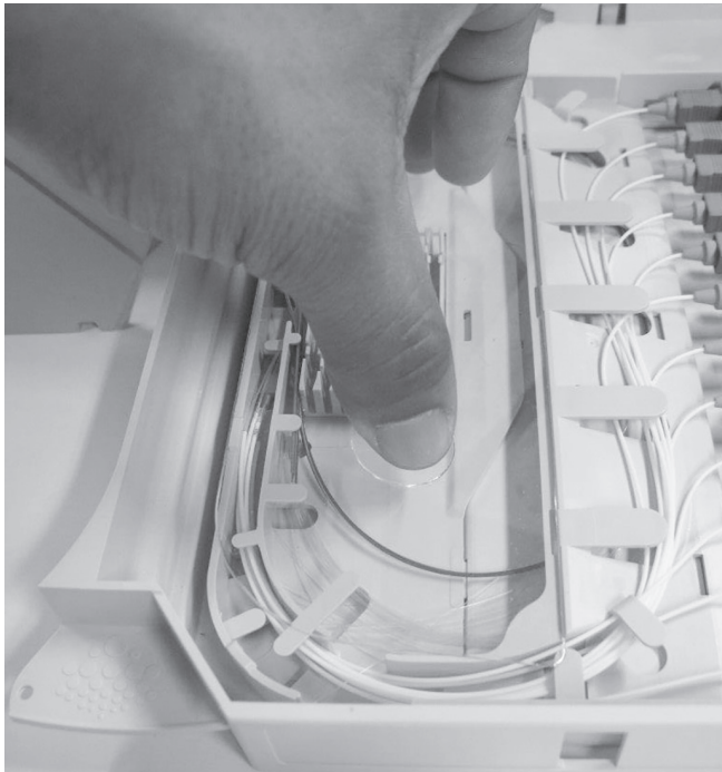
1.1 Remove plastic cover on splice island.
