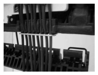
9.9 Put the drop cable behind the latch as shown.
