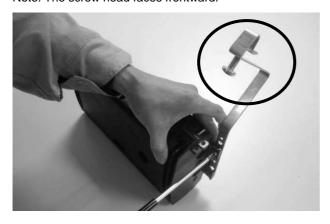
5.2 Secure the closure onto the strand wire firmly.
