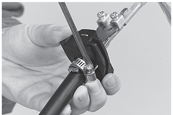
4.3.9 Install the cable retention device on the cable, tighten the hose clamp.
