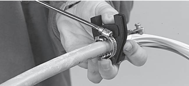
4.3.5 Install the cable retention device on the cable, tighten the hose clamp.
