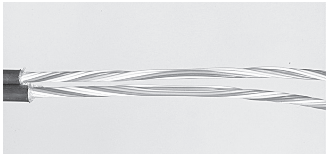
4.1.1 Make a window cut of 3.5 m. Cut the strength member at a distance of 50 mm.
