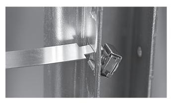
4.1.2 Install the cage nuts into the rack mounting uprights.
