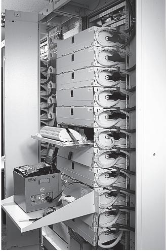
4.2.6 Place the splicing unit and necessary tools onto the table (max.  $25~{\rm kg}$ ) and prepare the to be spliced shelve according to the appropriate instruction.
