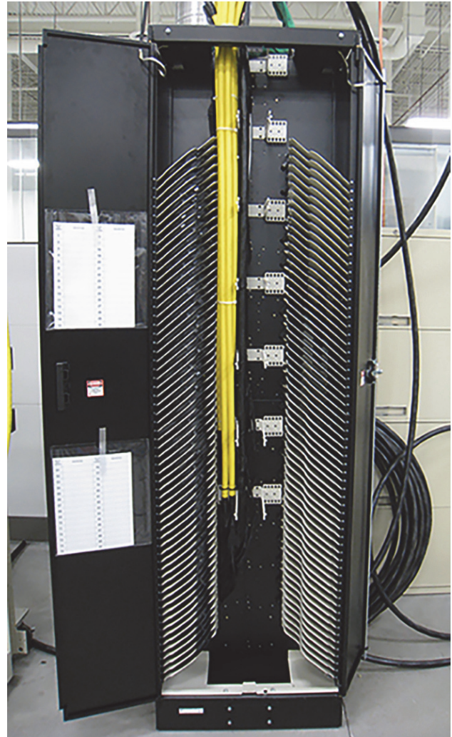
Figure 22. OMX Splice Cabinet With Slanted Shelves for Round Splice Trays
